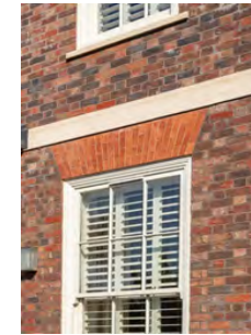
SIMILAR EXAMPLE OF PROPOSED FRONT ENTRANCE WITH STONE BAND COURSE AND GAUGED BRICK ARCHES
