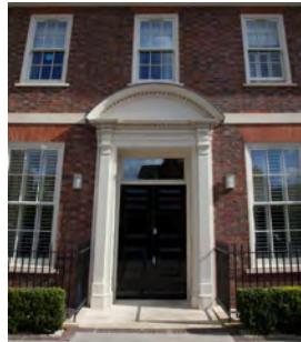
SIMILAR EXAMPLE OF PROPOSED FRONT ENTRANCE WITH STONE BAND COURSE AND GAUGED BRICK ARCHES
